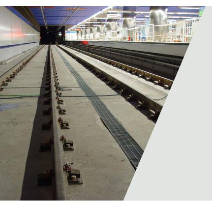
Pandrol's ADH System limits corrugation and vibration problems caused by the major dynamic forces generated by passing trains.
