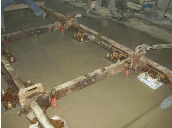
Figure 12: Direct concrete pour using either a construction shim or a slave plate
