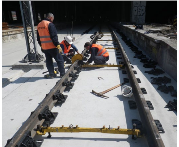
Figure 19: Clamping up in progress
