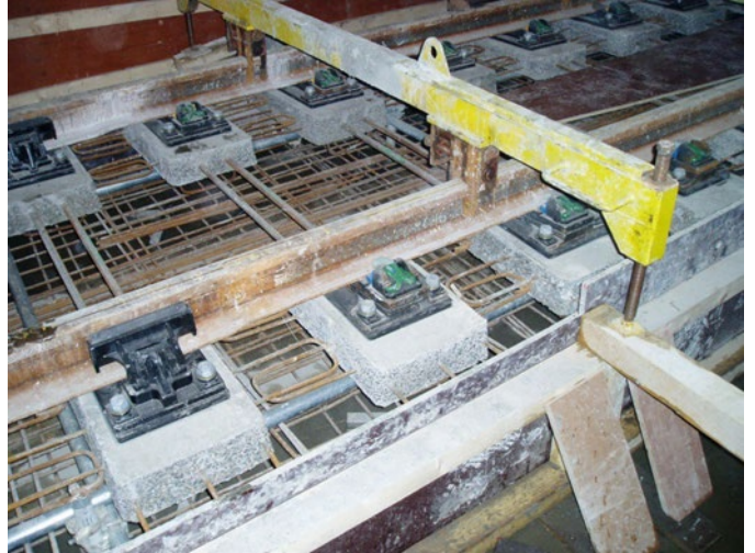
Figure 13: Direct concrete pour using a pre cast concrete element (block/sleeper)
