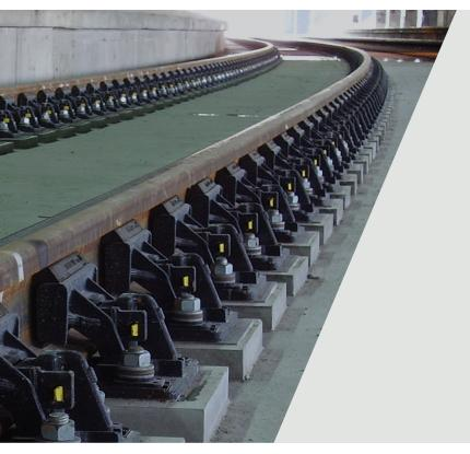
The Pandrol Vanguard rail fastening provides very low vertical stiffness, leading to high levels of vibration isolation at a much lower cost than alternatives such as floating slab. This makes it particularly useful for addressing ground-borne, or secondary, noise and vibration issues in sensitive urban environments.
