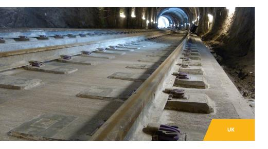
The Bowshank tunnel is fitted with track held firmly to retain long term alignment and allow high line speed on the sharply curved double track.
