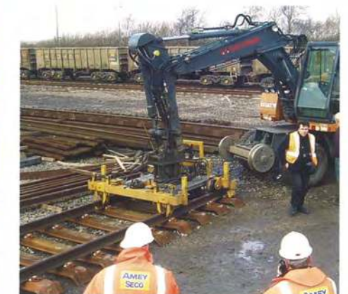
Figure 6 - Road-rail module clipping up FASTCLIP on steel sleepers.
