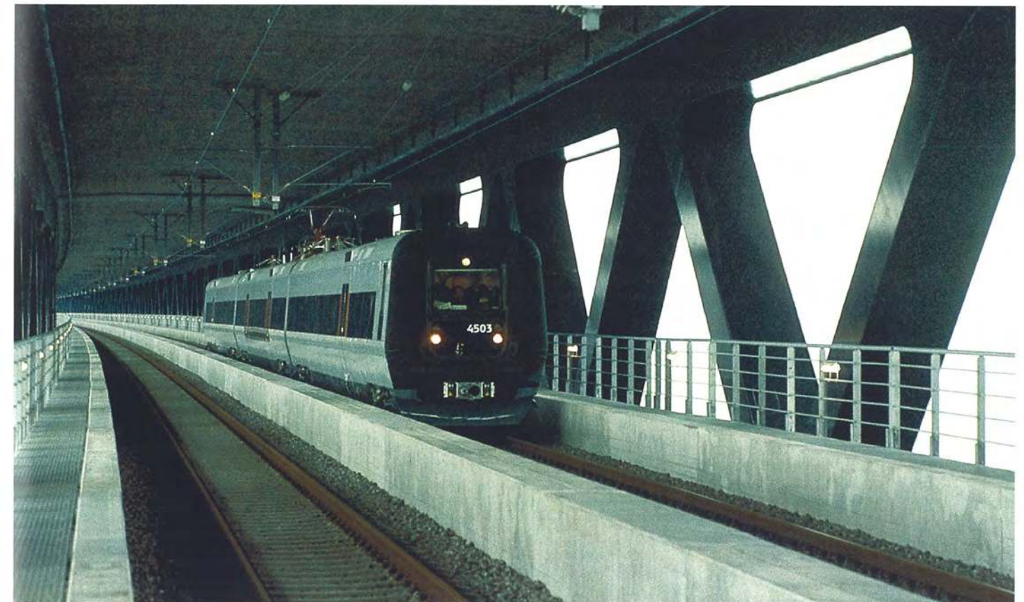
Train units run on the lower deck of the bridge.
