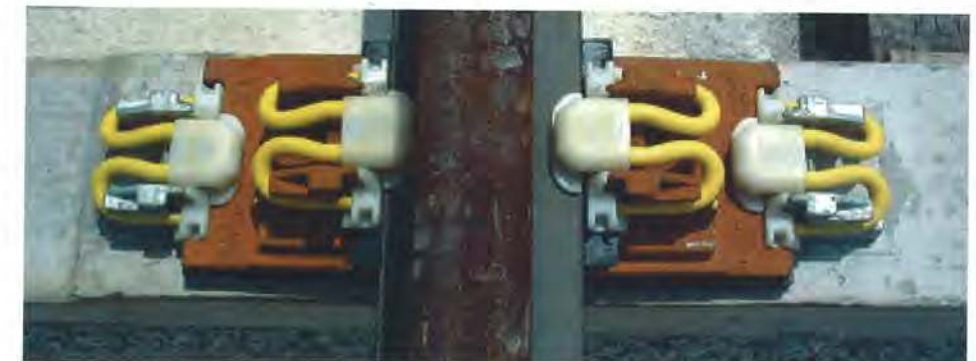
Figure 2b - Height Adjustable Assembly as installed on the NEL.
