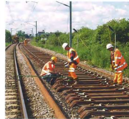
Figure 4 - FASTCLIP steel sleepers being laid by hand at Downham market.
