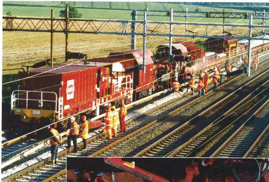
Above: Modified Fairmont Tamer P8-11 track laying machine.
