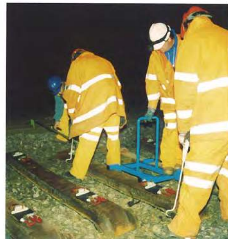
Figure 3 - FASTCLIP steel sleepers being laid by hand at Thetford.
