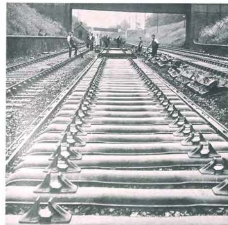
Figure 1 - Steel sleepers being installed during 1946.
