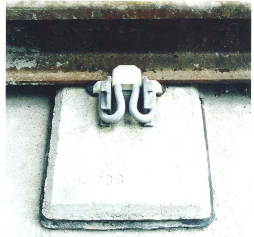
Rubber booted Sonnevile LVT blocks with FASTCLIP FC1501 rail fastenings.
