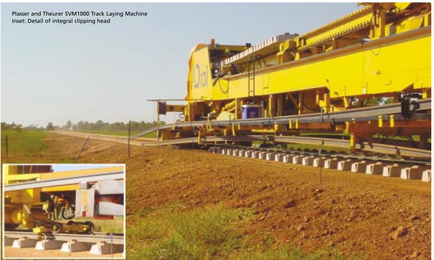
Concrete Sleeper pre-assembled with FASTCLIP fastenings
