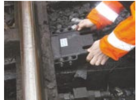
3. Offer Rotor Rail unit onto baseplate. Slide until rollers just touch switch blade.
