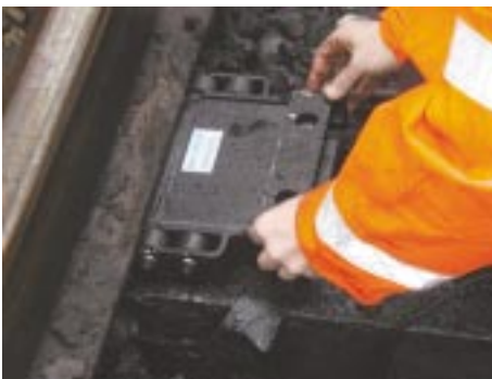
4. Place locking plates over holes ensuring serrations are facing down.
