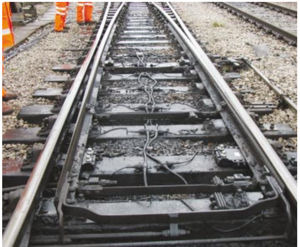
6. Once fitted, the entire site no longer requires greasing.
