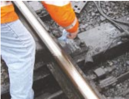
1. Remove AS screws and clean off excess grease from baseplate.
