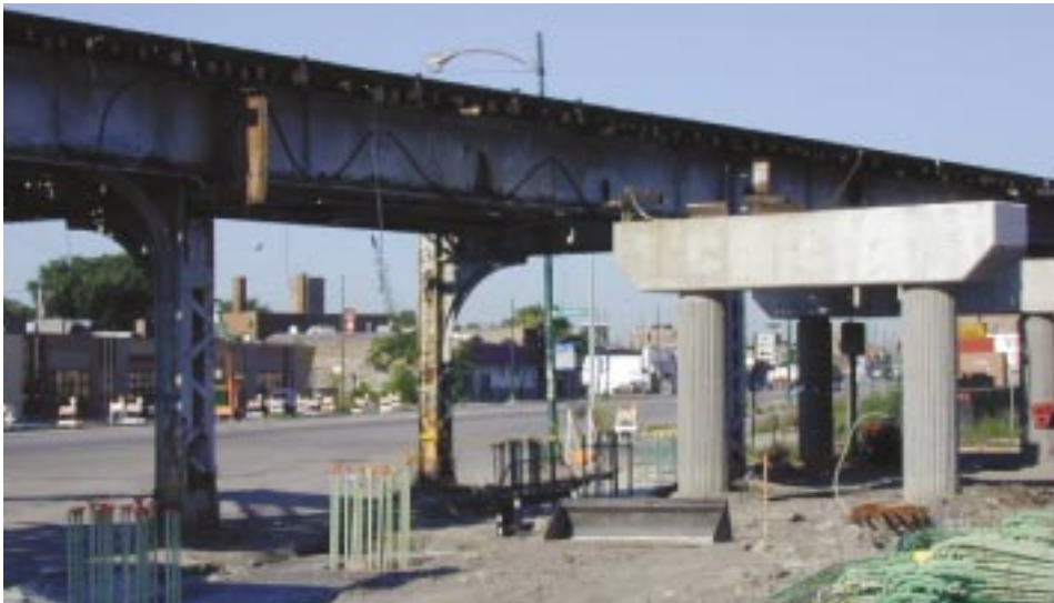
New concrete support structure
