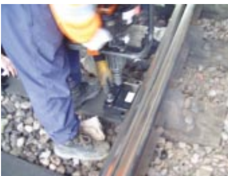
5. Replace screws in holes and tighten to correct torque. Note: Longer AS screws or Vortok Coils are recommended to be fitted.
