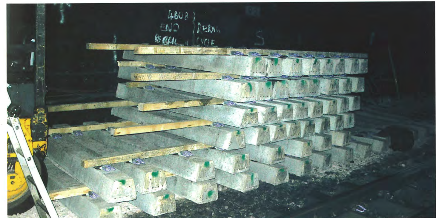
▲ G44 Sleepers pre-assembled with sheradised fastenings ready to be installed.
