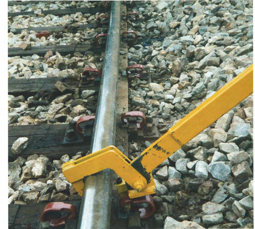
▲ Detail of K-Lock installation tool.
