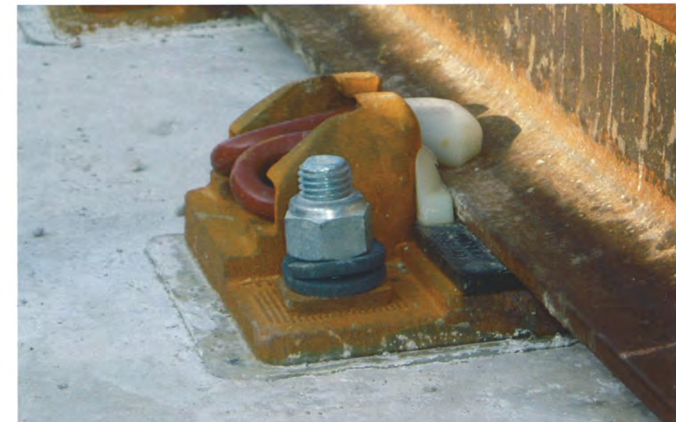
Middle: Locally manufactured plastic covers protect assemblies from the concrete fill.
