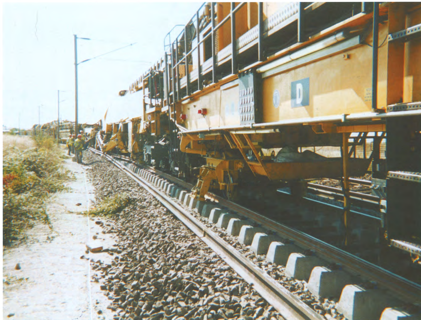
▲ Matisa Track Laying Machine.
