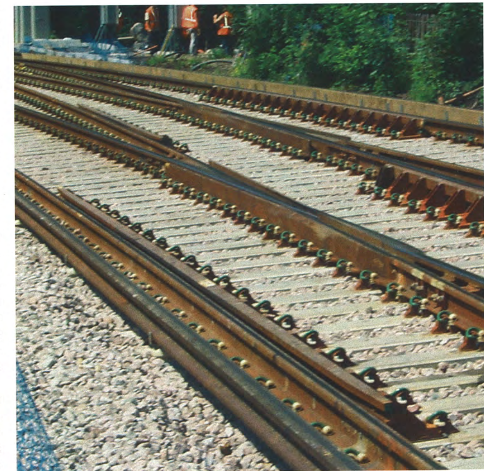
▲ e-PLUS Crossover at Shortlands Junction.
