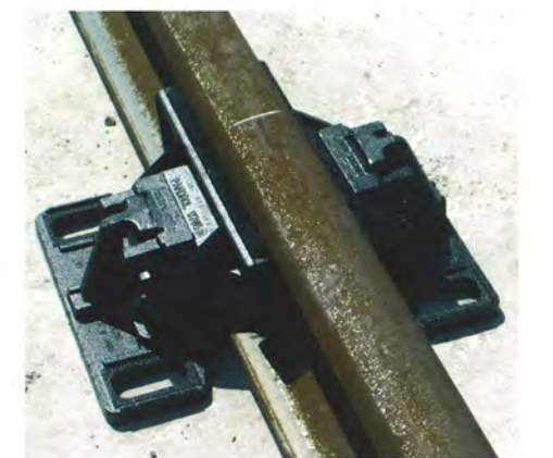
▲ VANGUARD assembled on rail. Photo by Mark Maher, RLE Senior Track Engineer.
