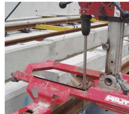
Drilling through to fix bolts
