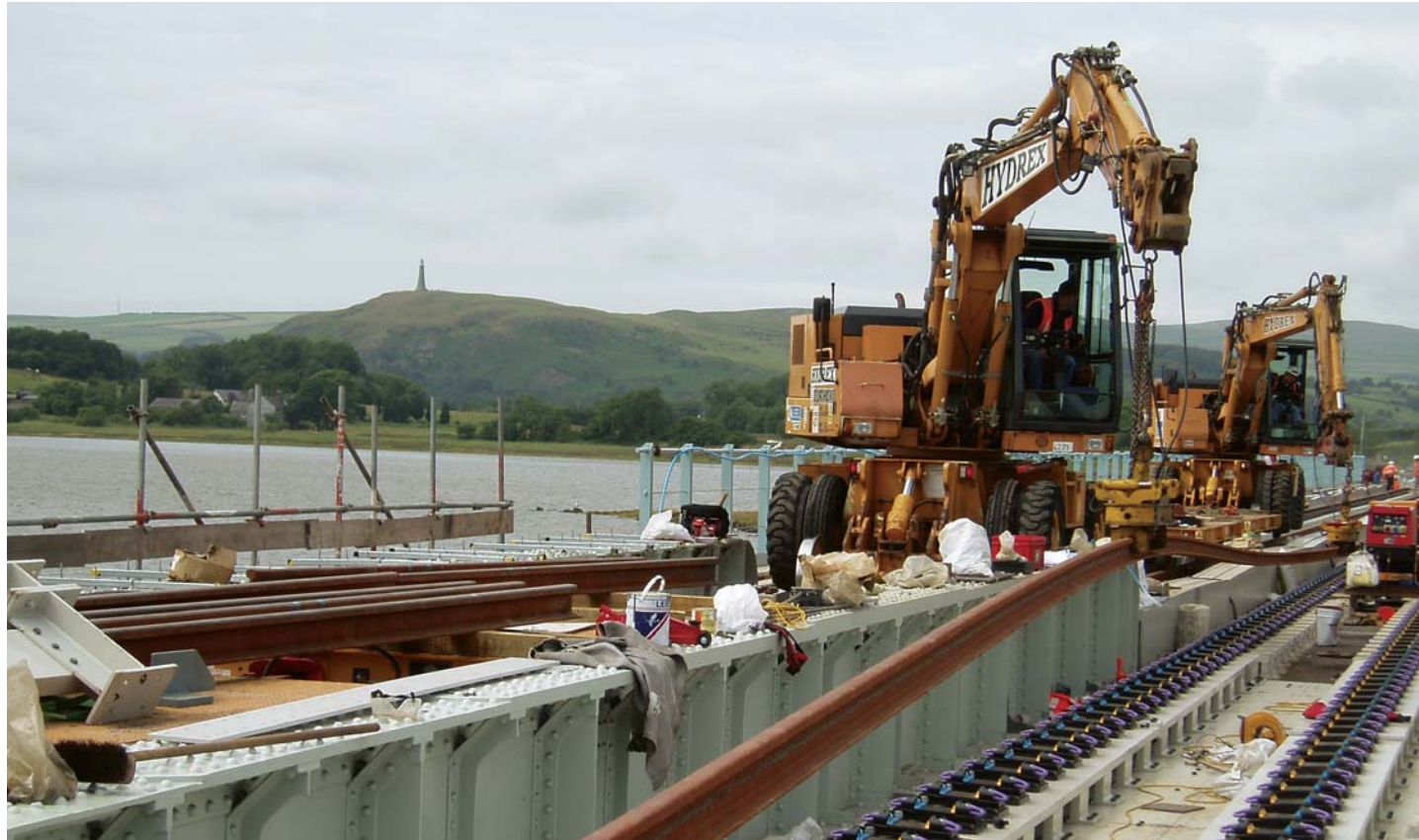
Threading Rail
