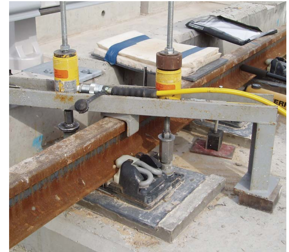
Proof load test on the anchor bolts on site
