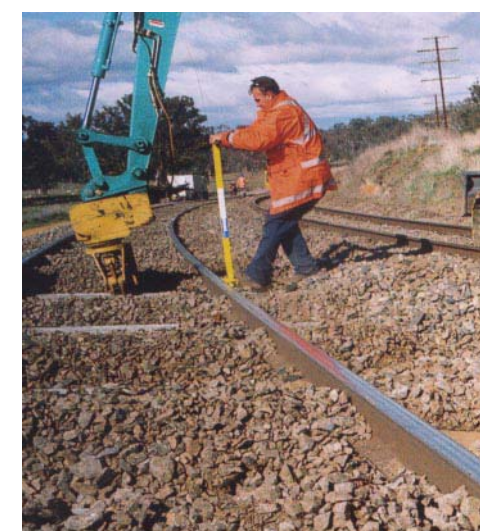
Mini Excavator used for laying out and installing sleepers
