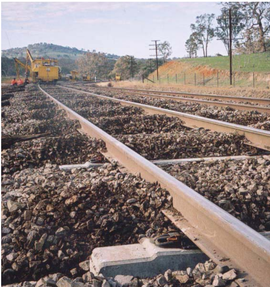
Installed sleepers prior to clipping up
