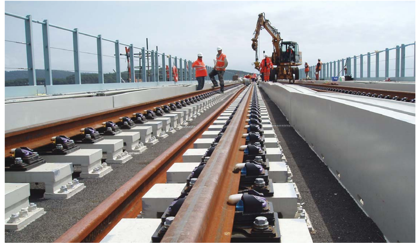
Lateral adjustment included in the PANDROL VIPA baseplates allows for accurate alignment of the finished track
