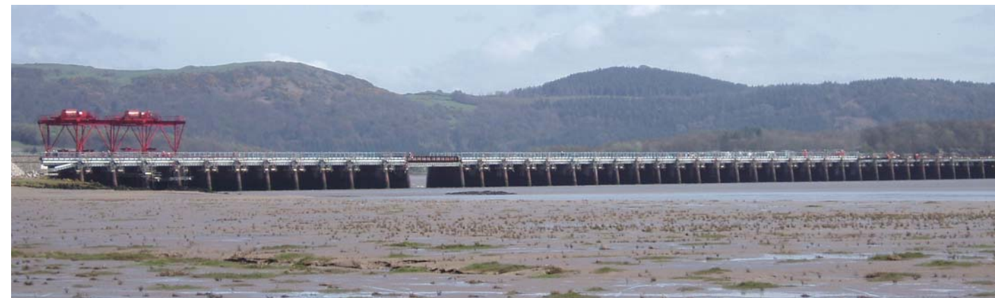
The Leven Viaduct
