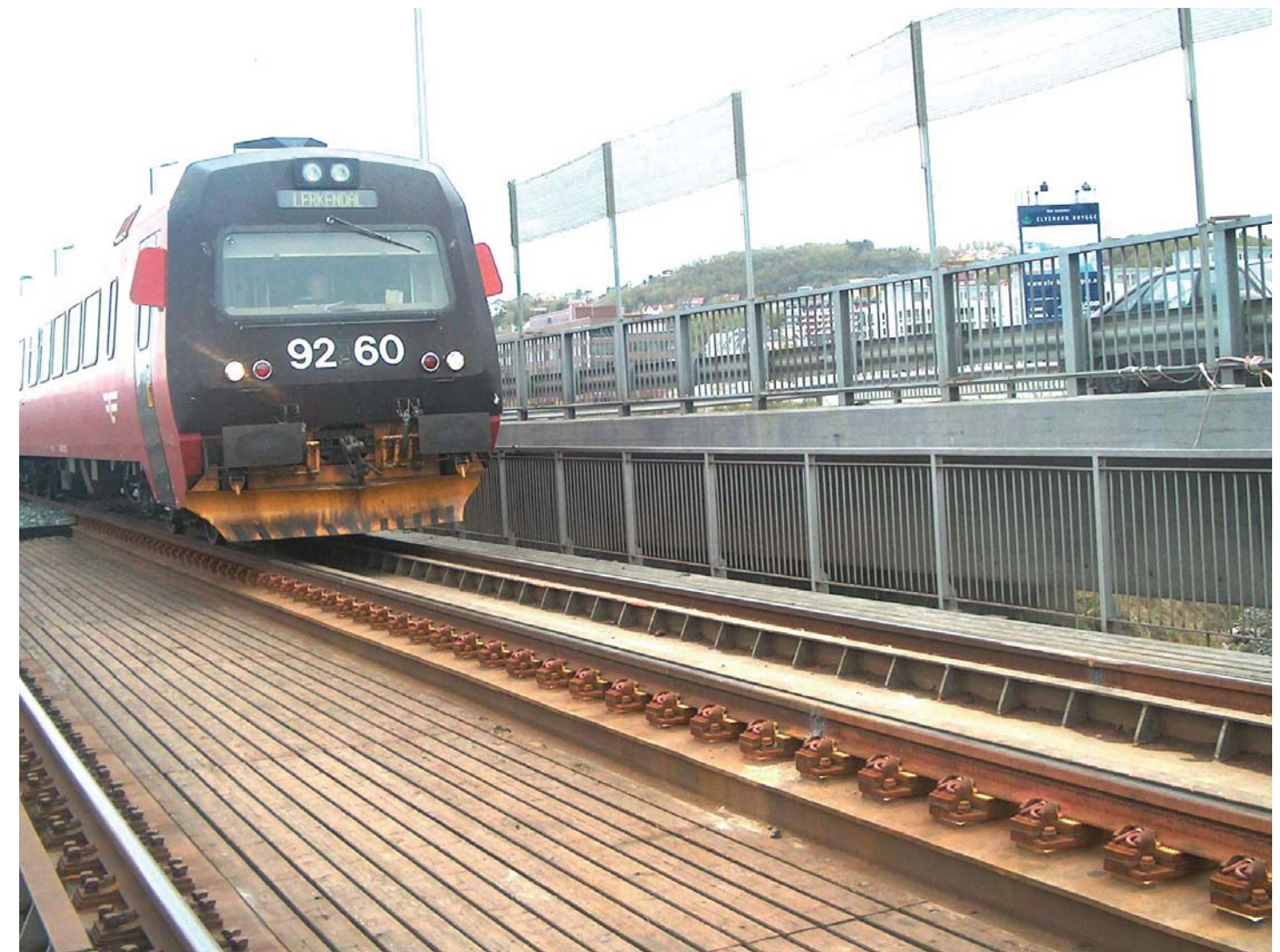
Commuter train BM92 passing over plate bridge
