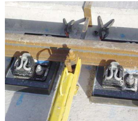
Formwork placed ready for pouring grout.
