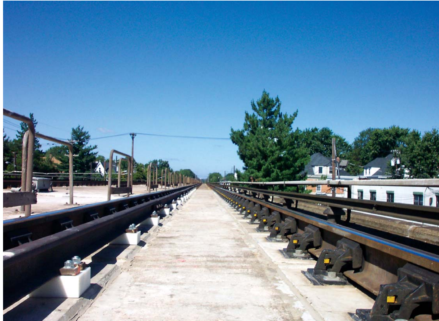
Completed PANGUARD Installation
