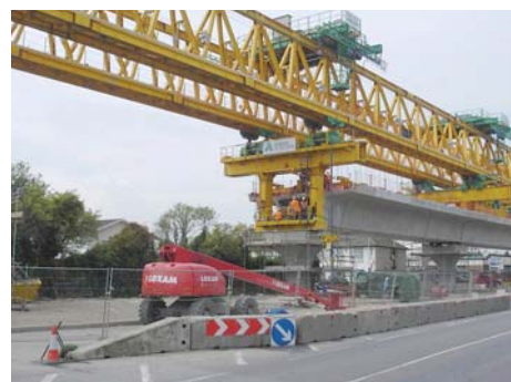
Gantry crane installing prefabricated viaduct segments
