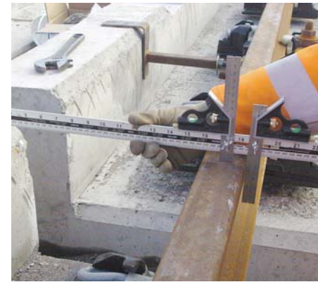
Track alignment checked prior to drilling for bolts.
