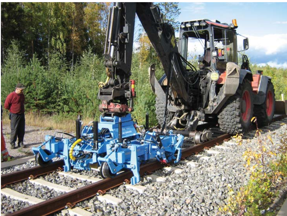
CD400 clip driver hydraulically powered by road/railer
