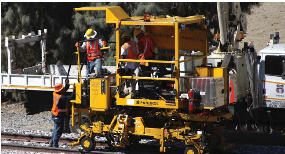
Rosenqvist CD500 hi-output clipping machine for Safelok 3
