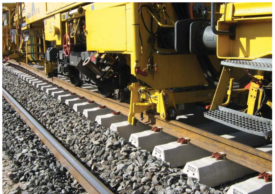
Clips correctly installed
