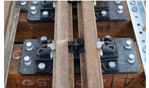
View of Dual Rail VIPA-SP Assembly with 3rd Rail Installed and 'e' clip fastening
