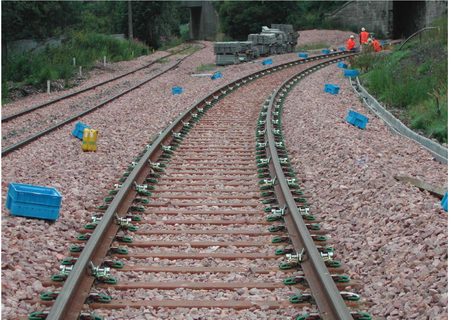
Vortok Stressing Rollers in track
