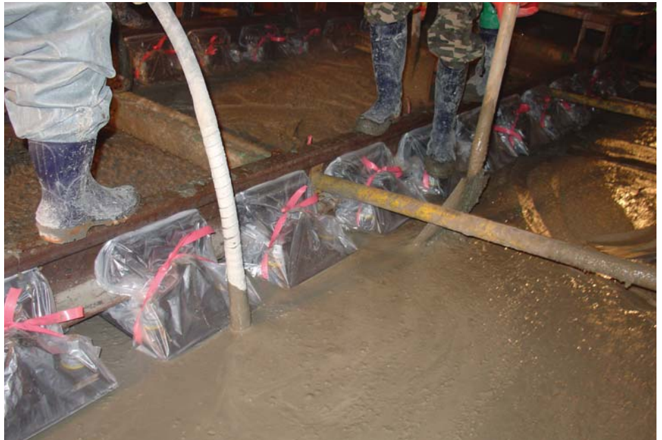
Concrete Slab being poured
