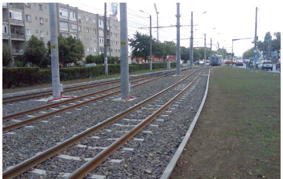
Modernised track with Pandrol Fastclip FD fastenings
