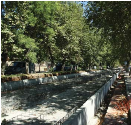
Preparation of base slab
