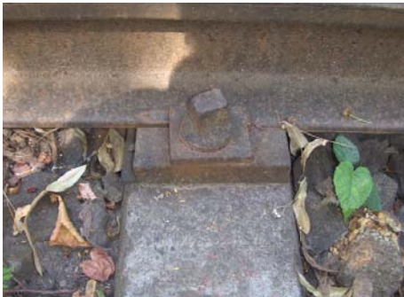
Original tracks fastened with screwspikes
