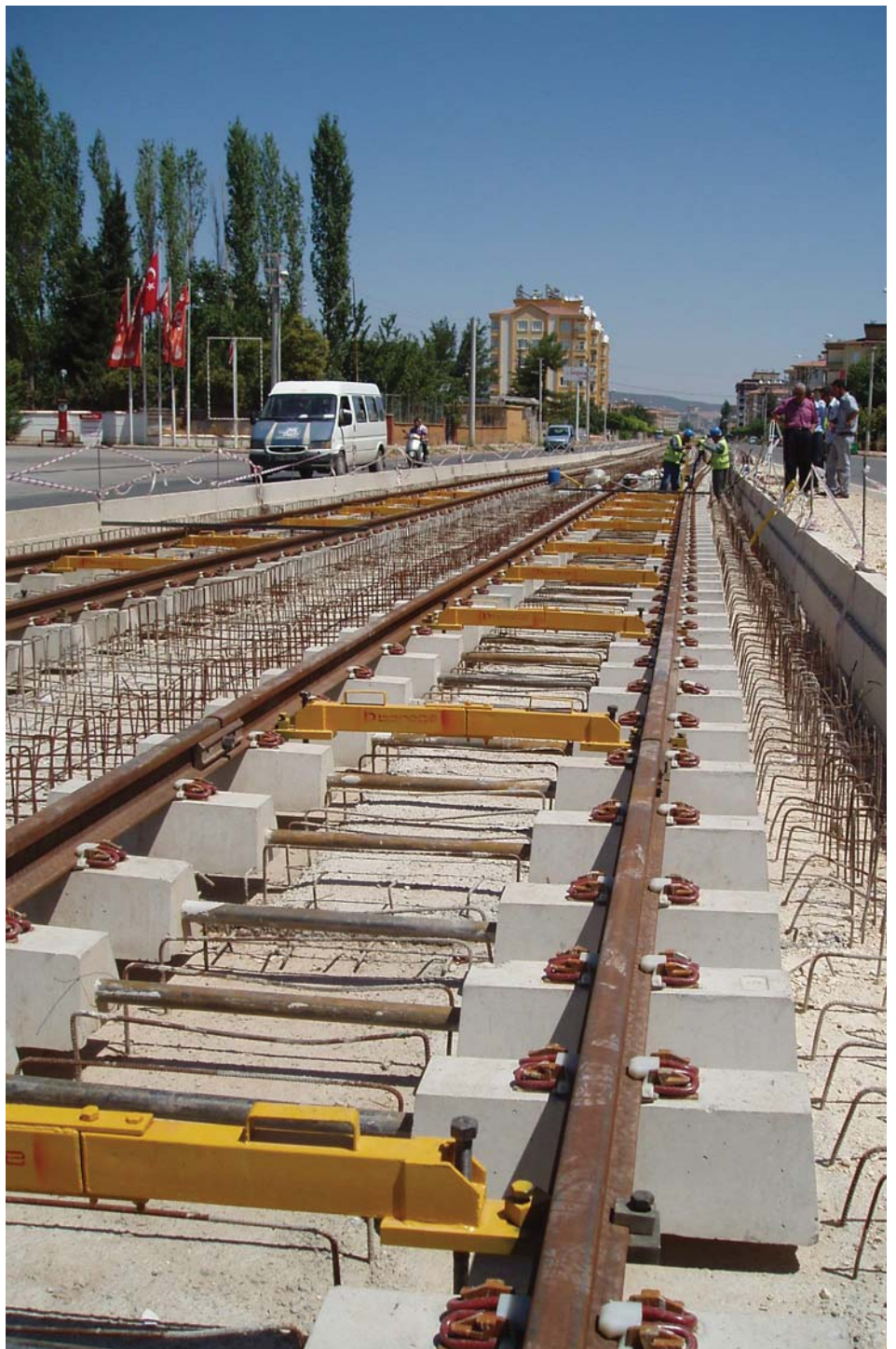
Twin-block sleepers with steel reinforcement prior to concrete pour
