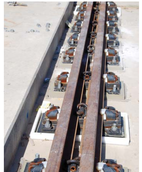
View of dual rail VIPA-SP assembly on lift up bridge span without 3rd Rail
