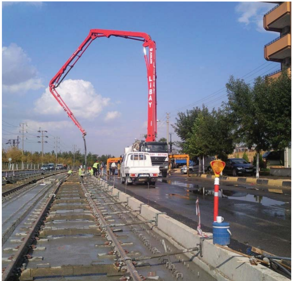
Concrete being poured to embed the sleepers
