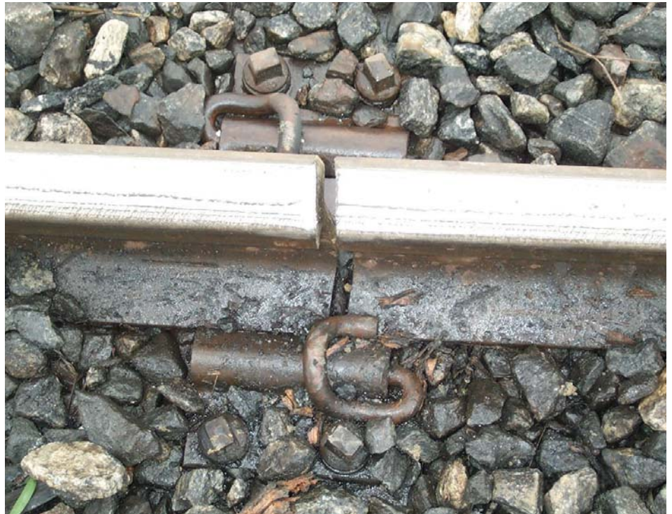
Figure 01 MRS 136 RE rail section pull-a-part
