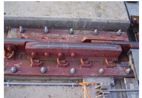
View of mitre joint
