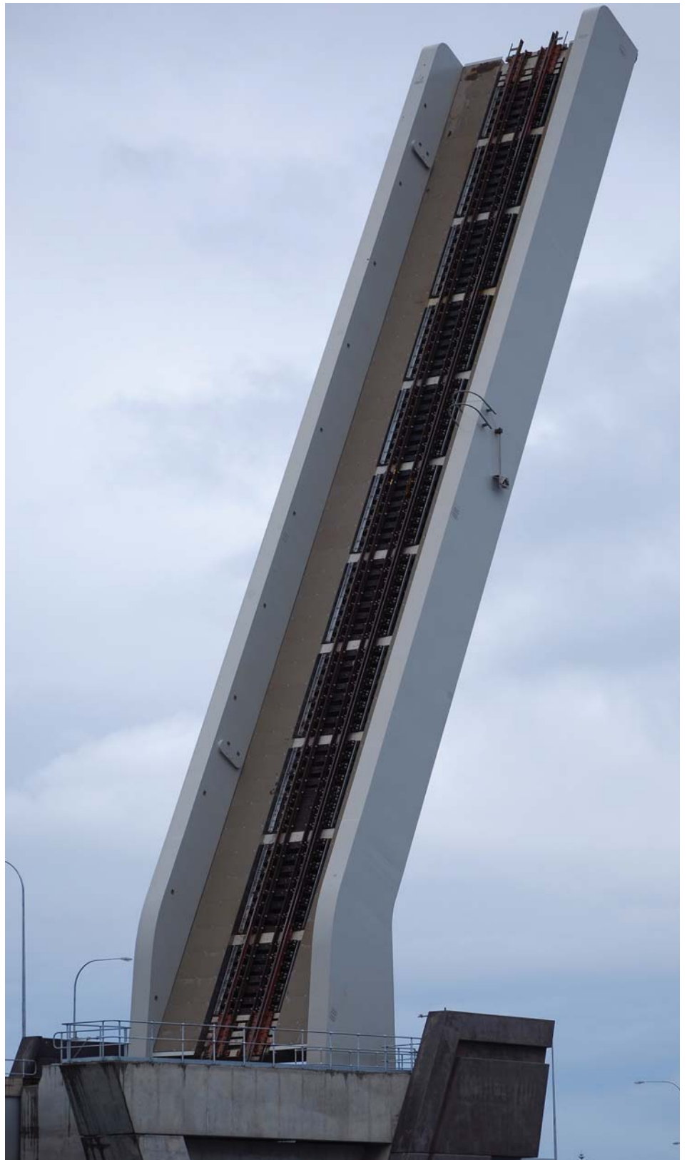
View of Bascule span
