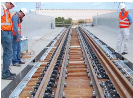
View of track on Bascule Bridge section
