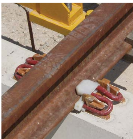
Rails are jugged to line and level
