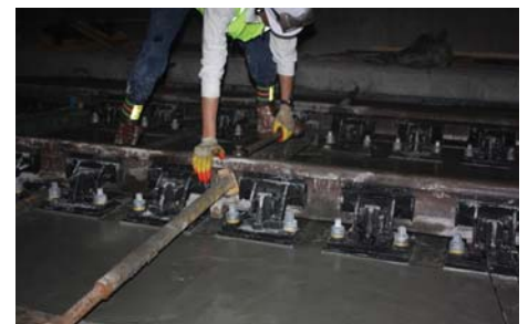
Track after concrete pour: making the final height adjustment
