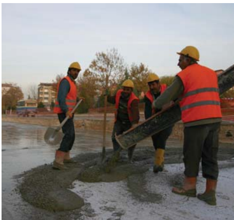
Even distribution of poured concrete
