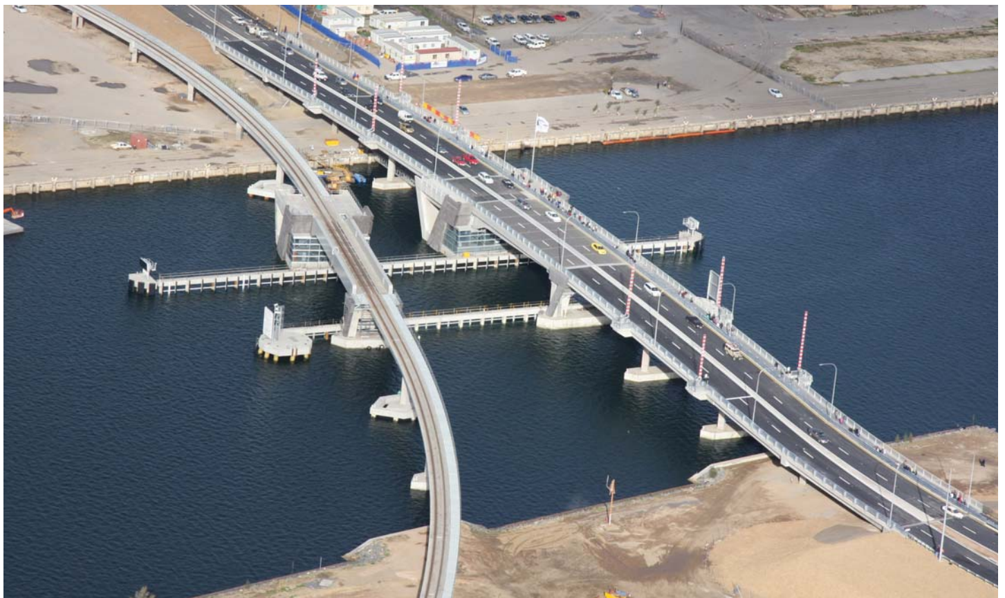
View of the Bascule Rail Bridge with the adjacent Bascule Road Bridge
