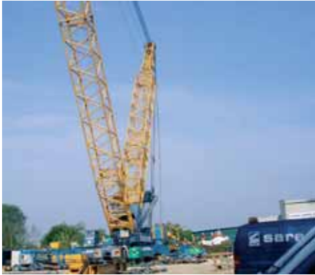
Crane prepares for bridge lift
