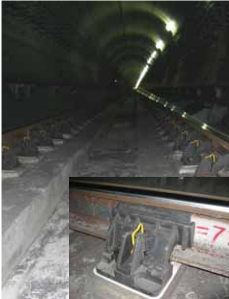
Figure 2(c) Finished VANGUARD installed on Beijing Subway Line 5
