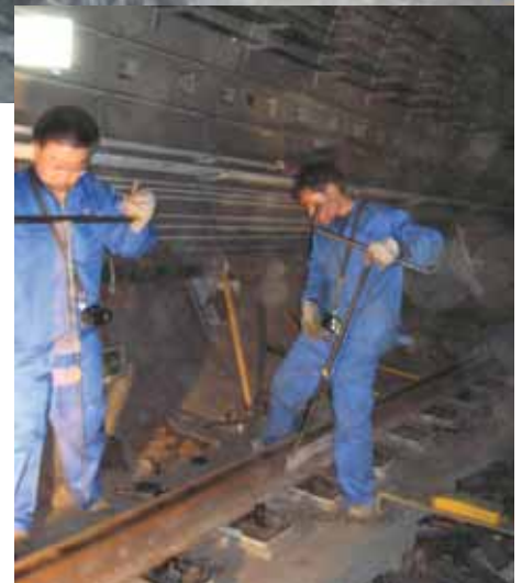
Figure 2(a) Delivery of VANGUARD components and removal of existing baseplate on Beijing Subway Line 5
