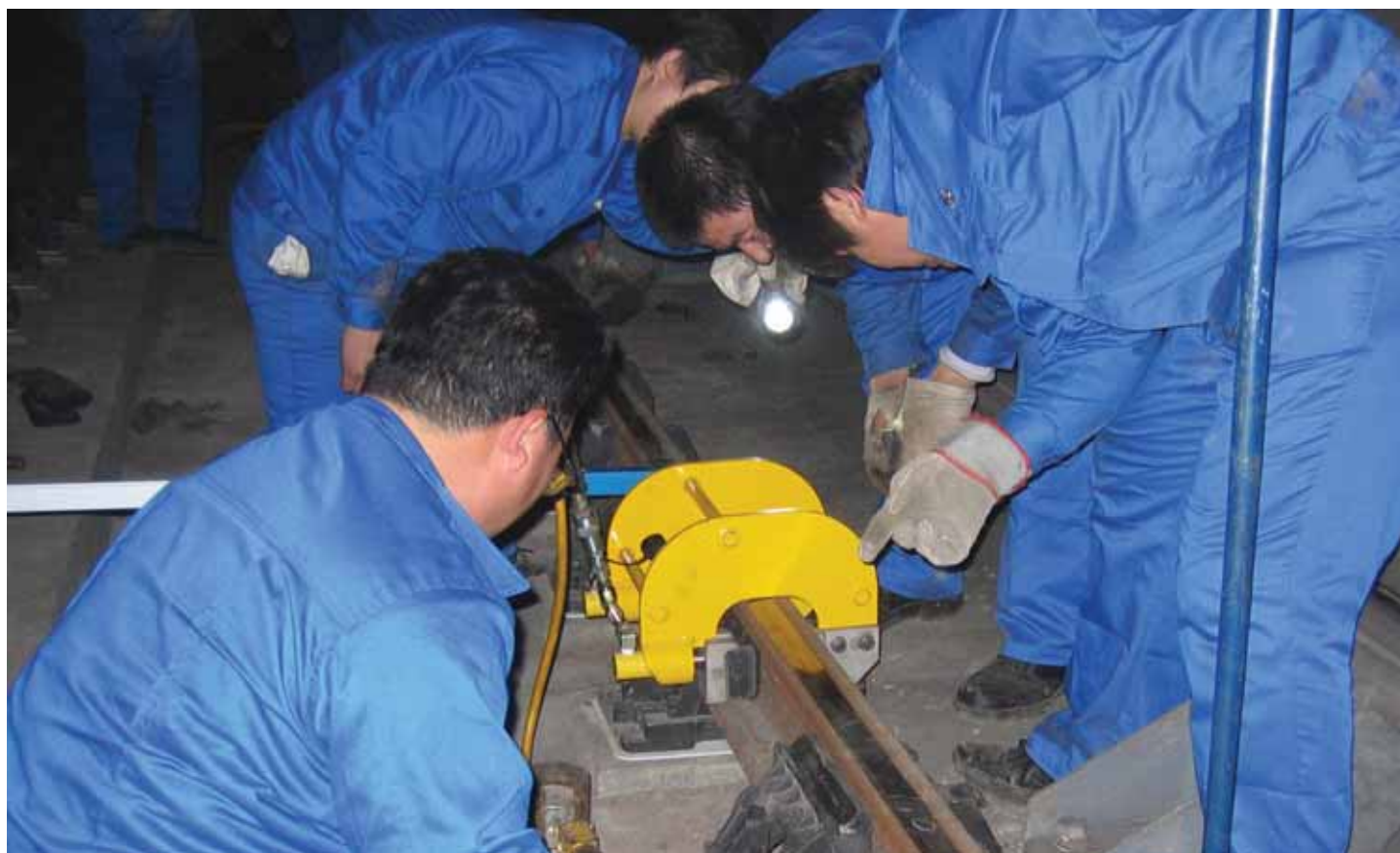
Figure 2(b) VANGUARD clamping
