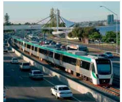
Finished track – Perth-Mandurah route
