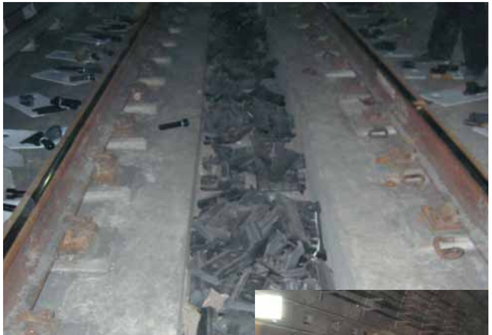
Figure 2(a) Delivery of VANGUARD components and removal of existing baseplate on Beijing Subway Line 5
