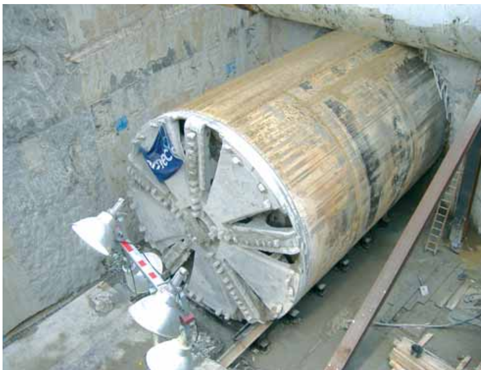
Woolwich – Arsenal tunnel breakthrough
