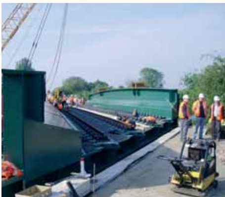
Bridge ready for final track adjustments after craning
