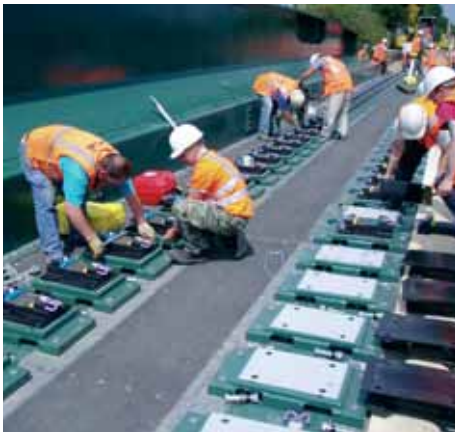
Inserting shims to achieve railhead design height
