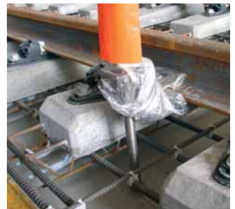
Sleepers raised with spindles after iron rods assembled beneath
