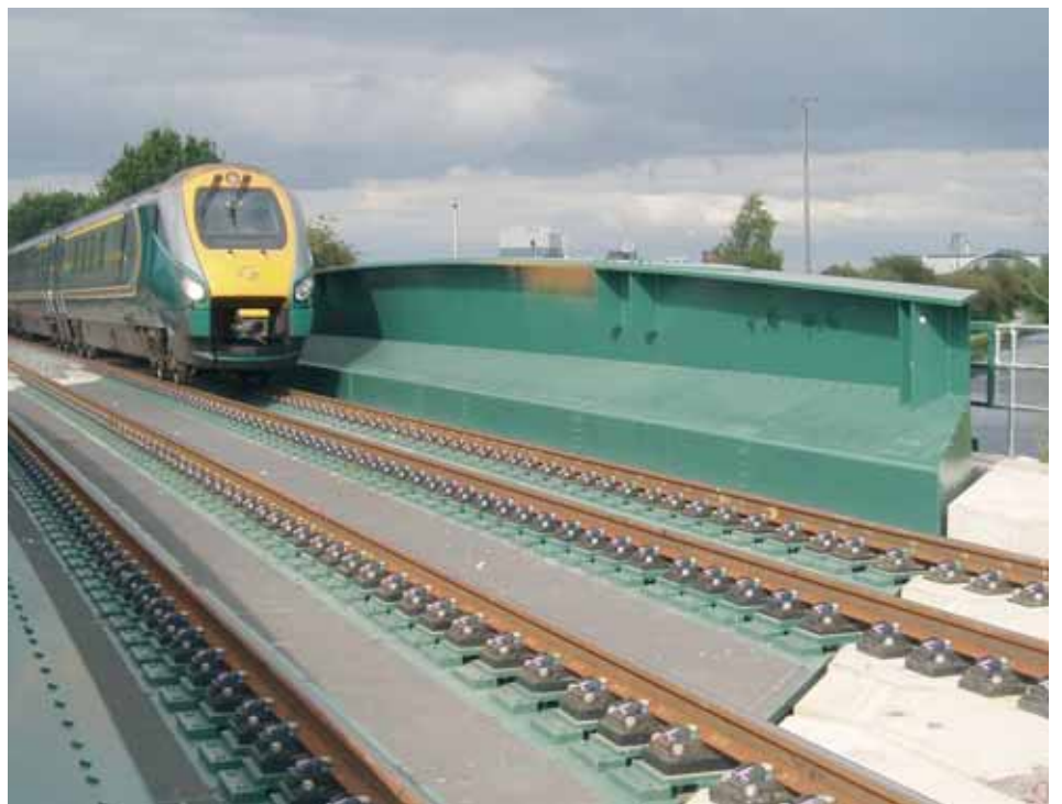
Completed track at Selby
