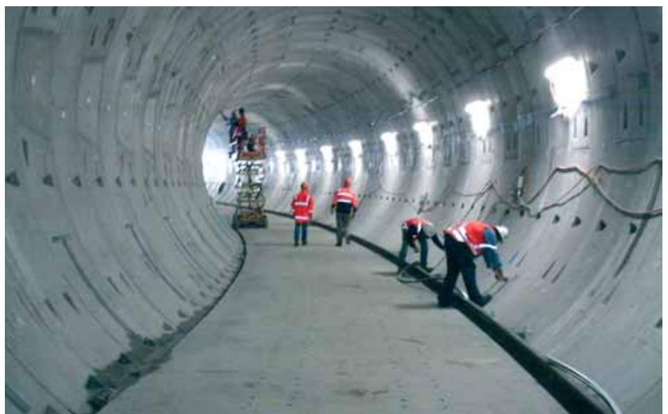
Bored tunnel under the Perth CBD
