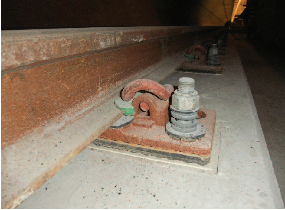
PANDROL Resilient baseplate assembly
