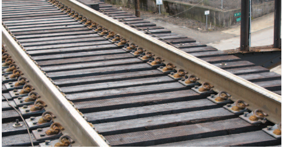
VICTOR baseplates with PANDROL brand e-Clips
