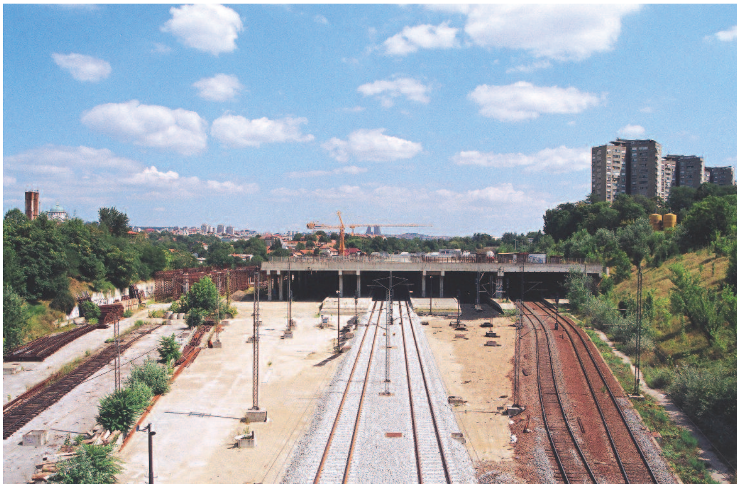
Overview of the construction area
