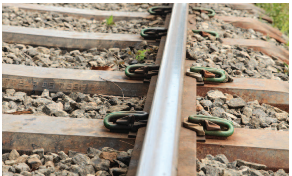
Finished track after rehabilitation
