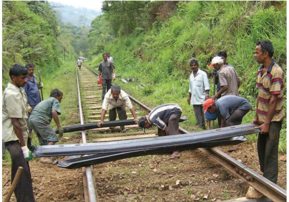
Steel sleepers replacing life expired timber sleepers
