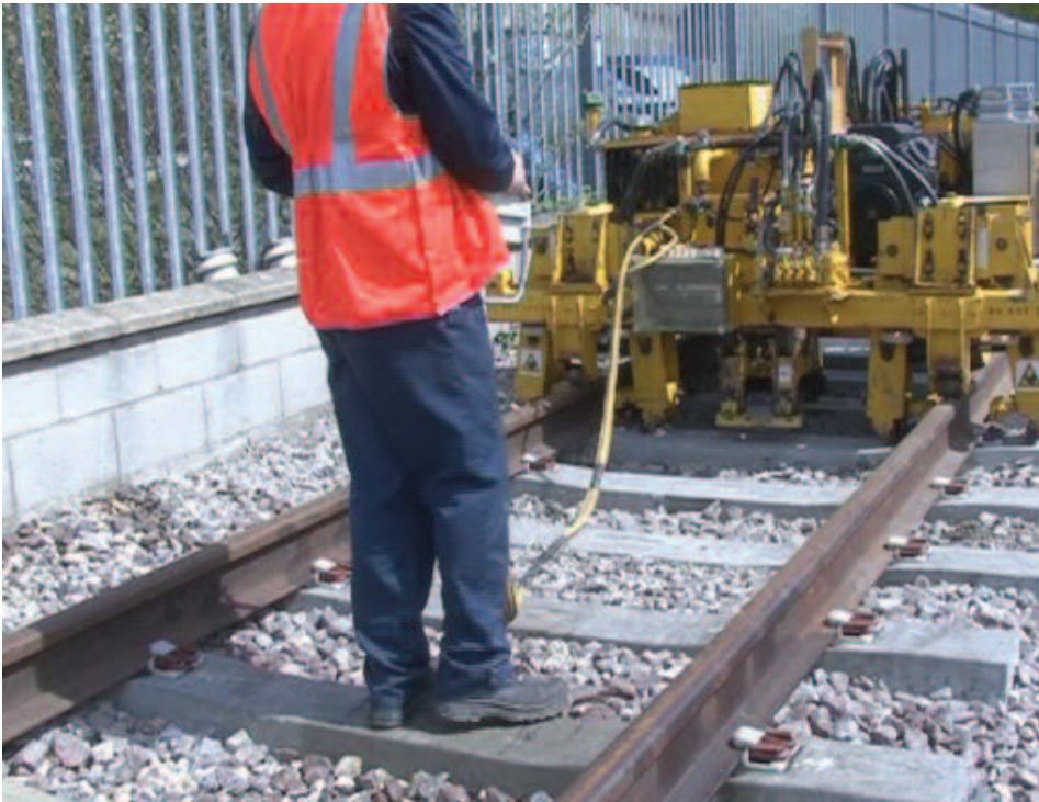
PANDROL MARK1V FASTCLIP installation machine
