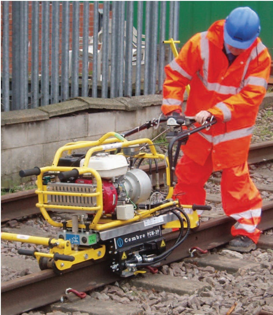
Installing Re clips using a Cembre installation machine
