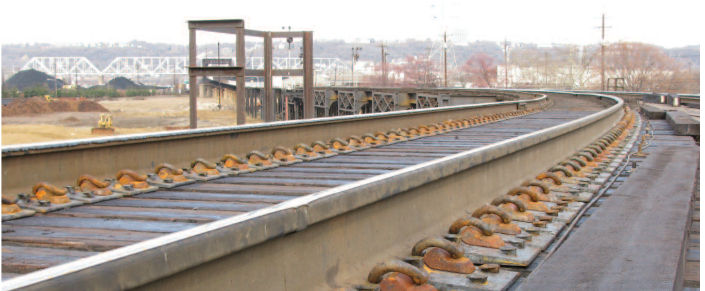
VICTOR baseplates with PANDROL FASTCLIP
