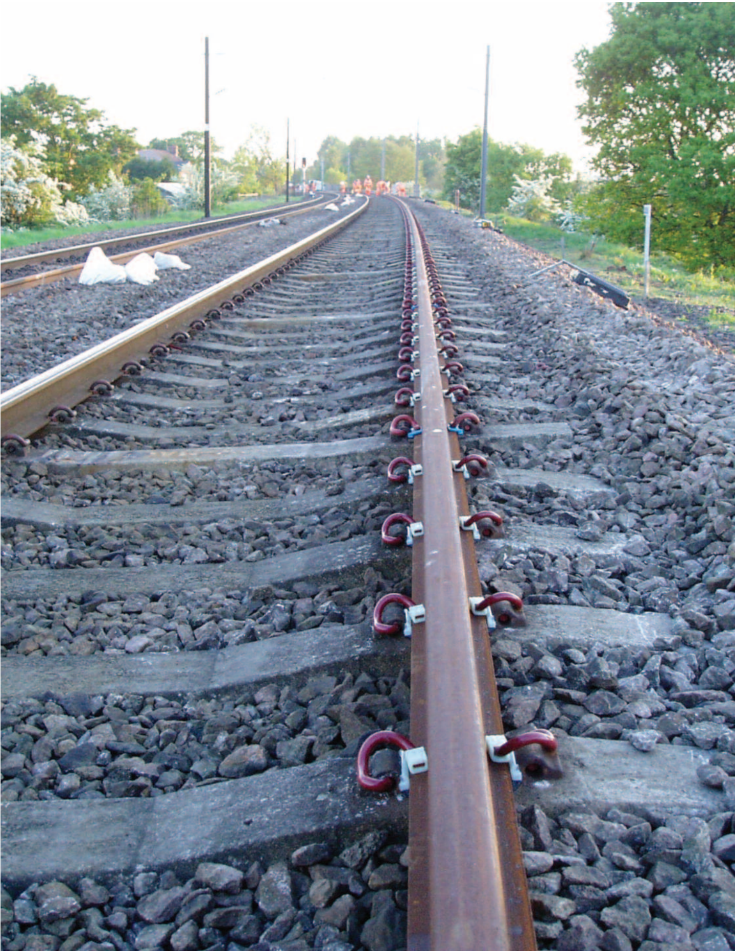
Completed track on Network Rail, UK
