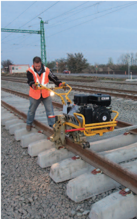
Rosenqvist CD200 installation machine for FASTCLIP
