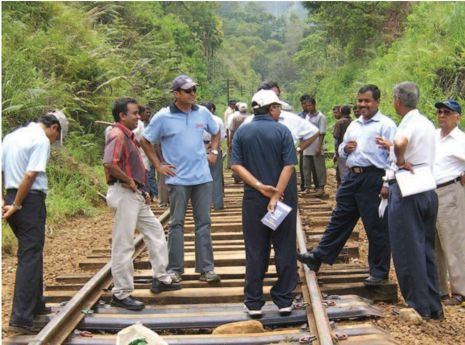
Initial trial installation
