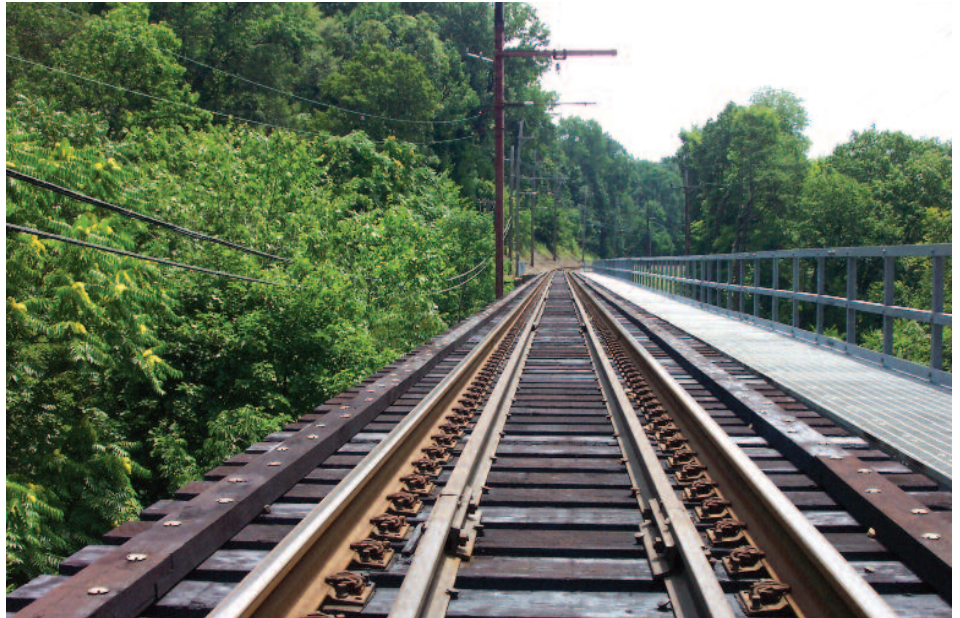
VICTOR baseplates with PANDROL FASTCLIP
