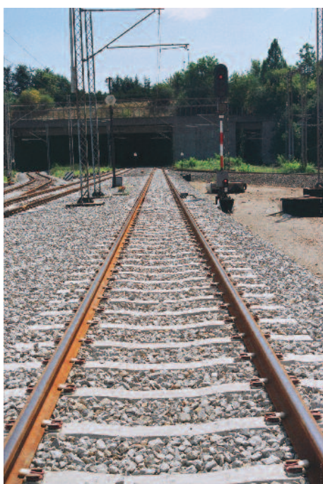
PANDROL FASTCLIP FE in ballasted track
