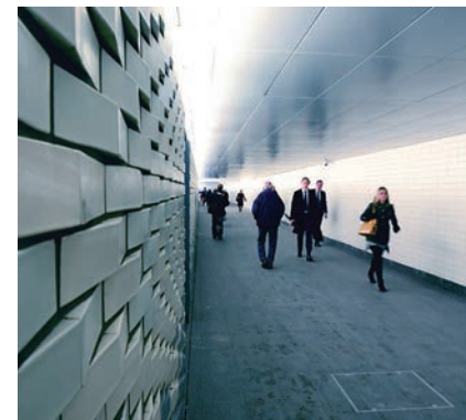
The interior of the pedestrian subway with high surface quality finishes and vibration attenuation provided by Pandrol VIPA-SP baseplates supporting the track overhead
