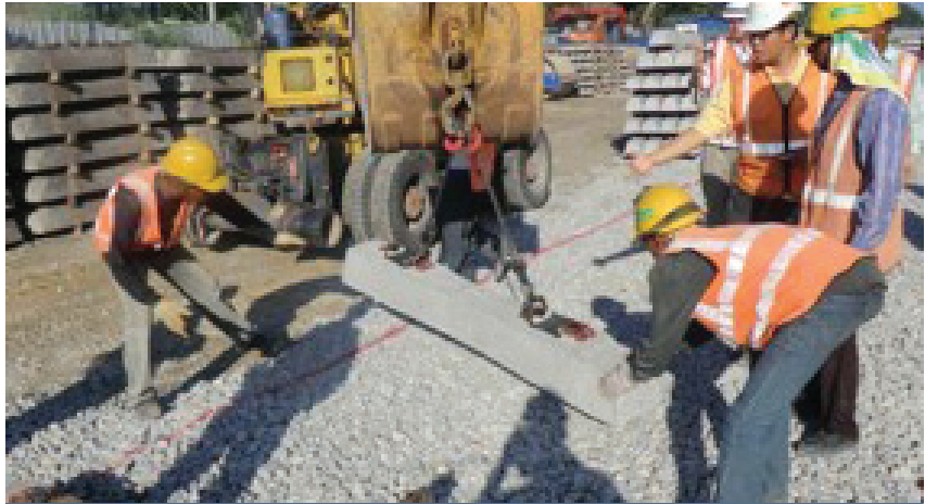
Installation of sleepers at site
