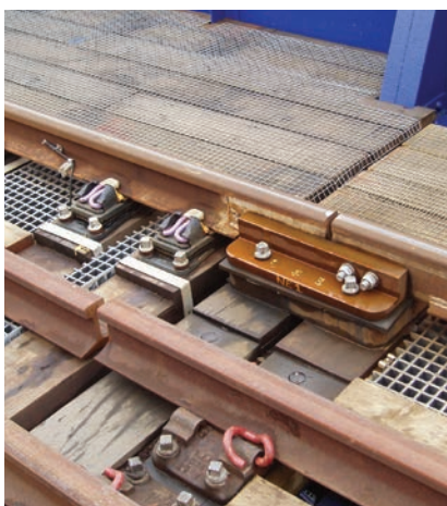
Detail of lifting joint and receiving blocks
