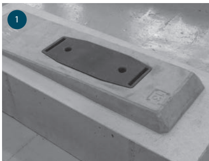
1 Plastic sub-plate and anchor inserts cast into pre-cast element.
