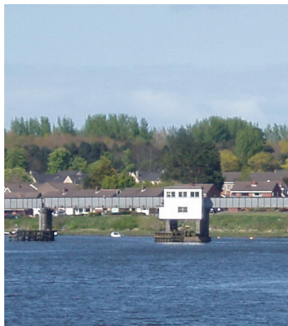
Bridge after refurbishment, April 2013
