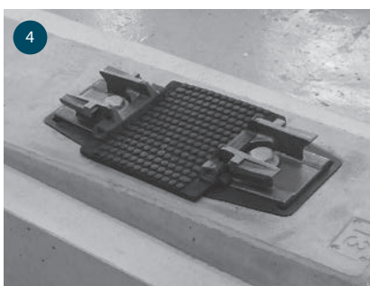
4 Rail pad and post insulators installed in the rail seat.
