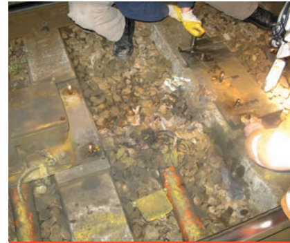
Drilling the sleepers
