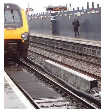
The concrete 'lid' of the subway after installation and opening to traffic
