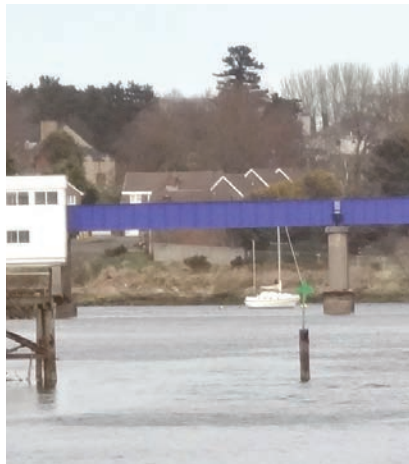
Bridge before the refurbishment, April 2012
