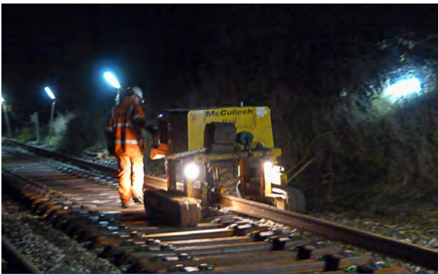
Rail threading using a McCulloch TRT
