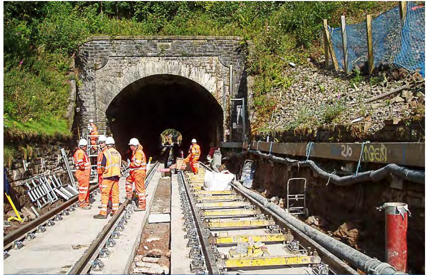
The southern portal
