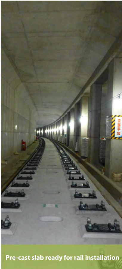
Clips ready for rail installation
