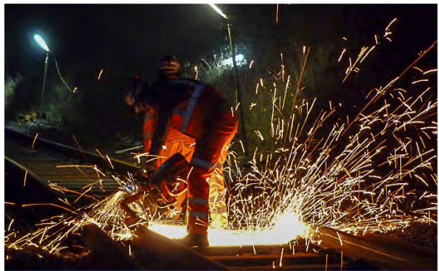
Cutting the rails with abrasive disc
