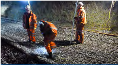
Painting a guidance line on the ballast
