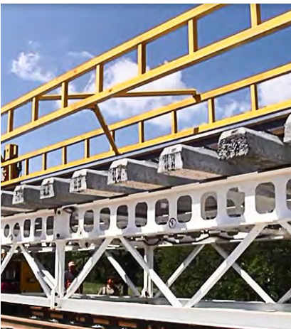
Panel Transporter Shuttle and Panel Layer
