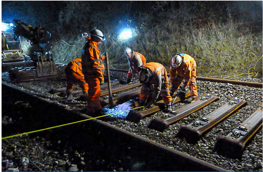
Checking the alignment from fixed survey points
