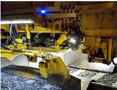
Ballast profile blades remove excess ballast
