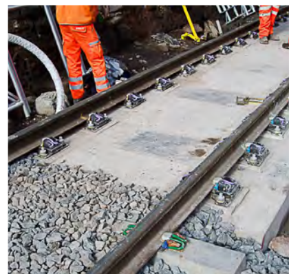
Transition between ballast and slab at the Southern portal
