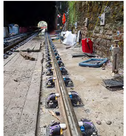
VIPA-SP with anchor screws into inserts
