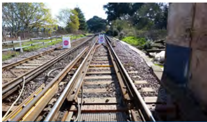
Transition and guard rail assembly on the approach side of the bridge
