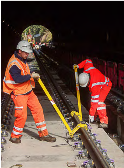
Inserting the clips with hand-tools
