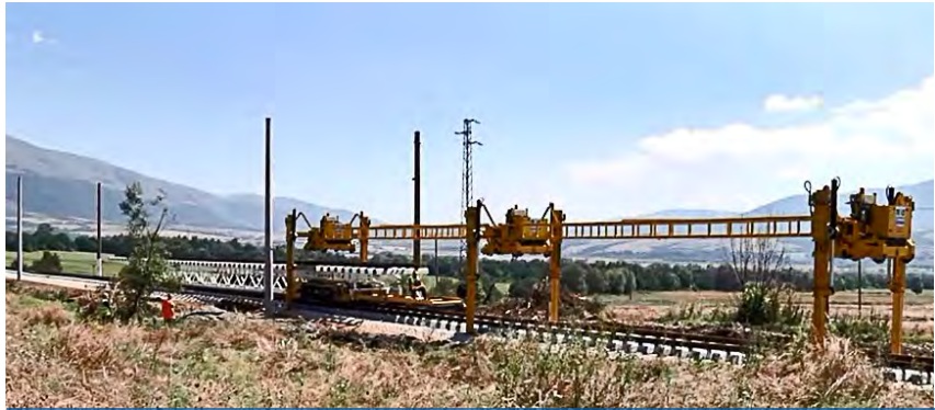
Panel Transporter Shuttle and Panel Layer
