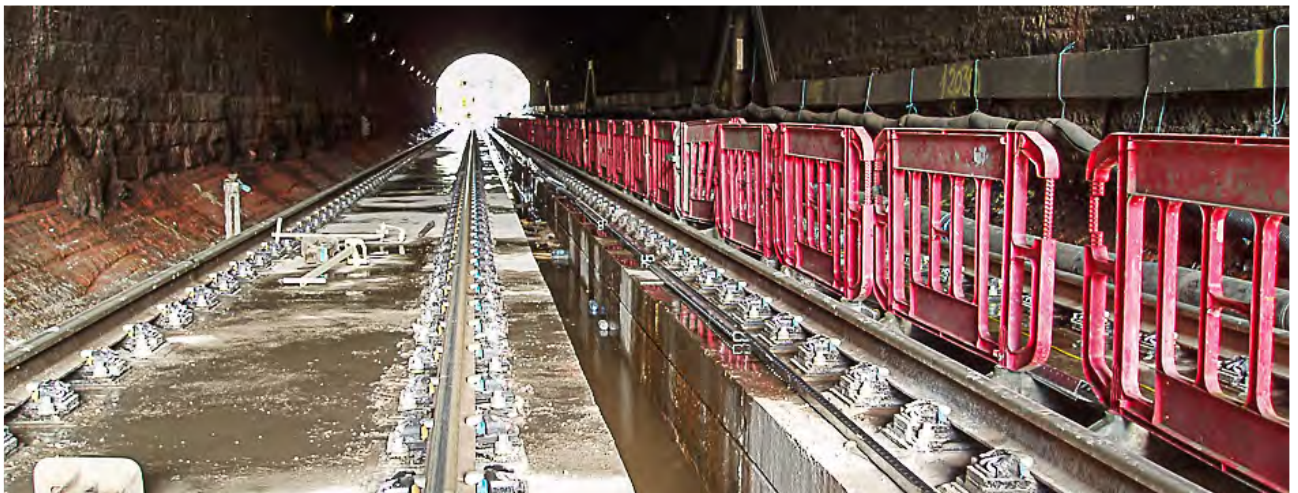
Completed track on the down line looking northwards
