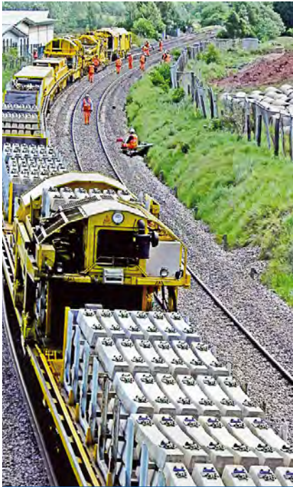
The sleeper delivery gantry in the foreground with the main sleeper exchange gantry in the background
