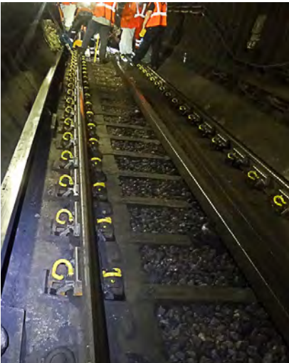
Holland Park installation
