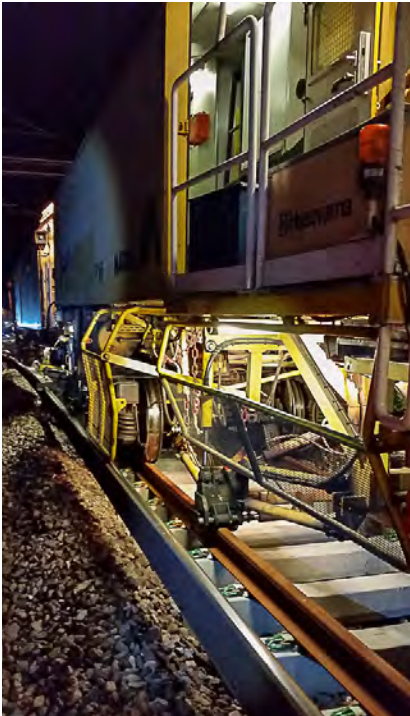
Threading in the new rails
