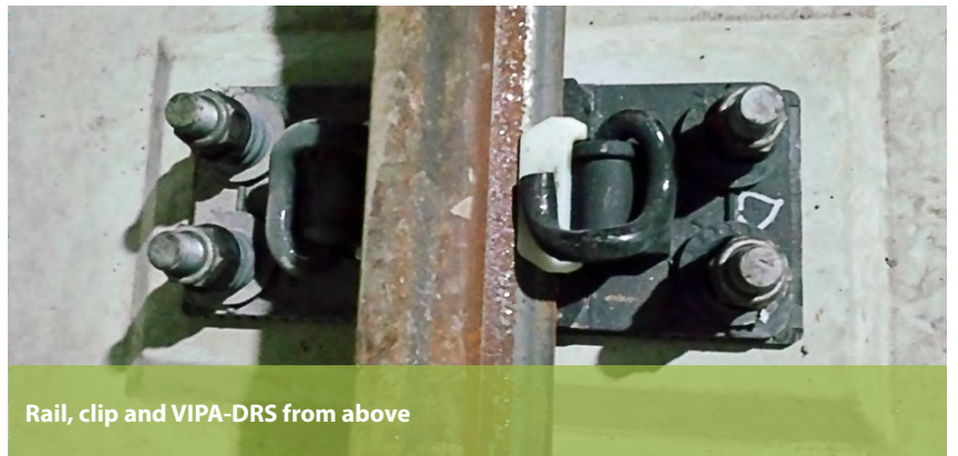
Clips ready for rail installation
