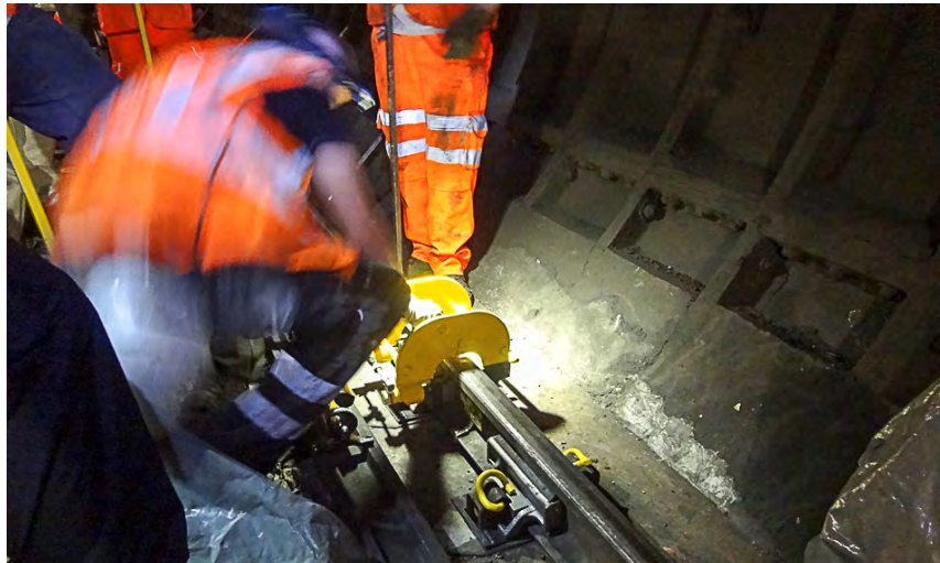
Hydraulic tool compresses the rubber components
