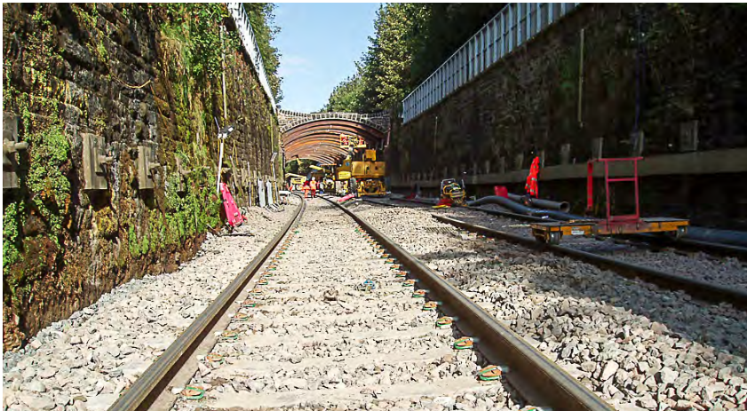
Ballast track: G44 concrete sleepers under the refurbished 'Flying Arches'
