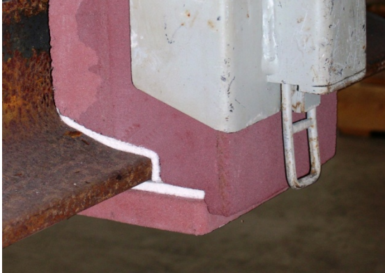
Figure 34: Check the Briquette fits
