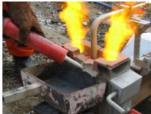
Figure 22: Luting paste application
