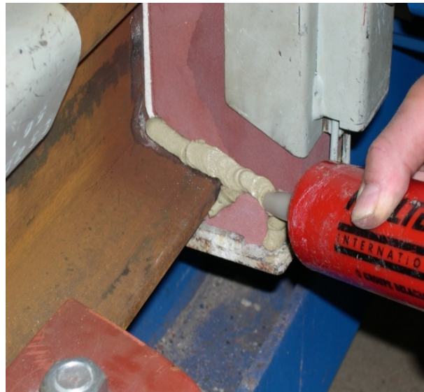
Figure 14: Application of luting paste
