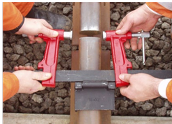
Figure 2: Position Clamp Assembly
