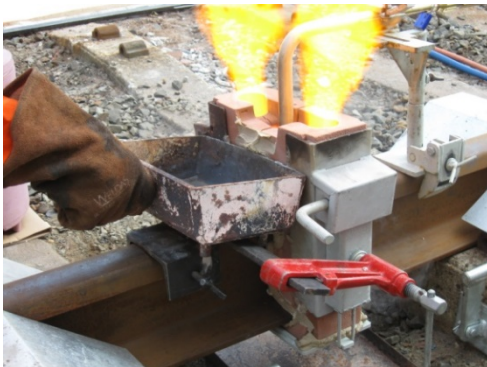
Figure 21: Attaching the slag bowl
