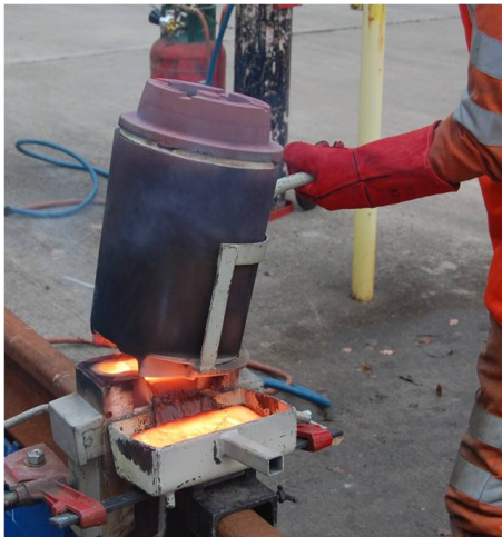
Figure 28: Crucible Removal
