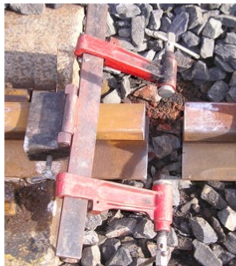
Figure 31: Positioning the Clamp
