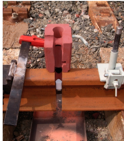
Figure 15: Correctly Fitted Mould
