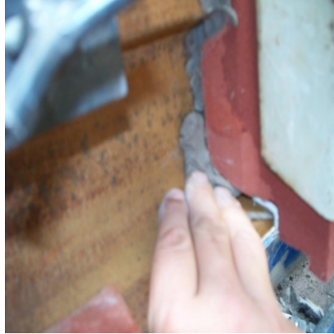
Figure 53: Correct method for applying the Pate A Lute
