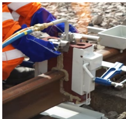
Figure 3: Self-Centring Burner
