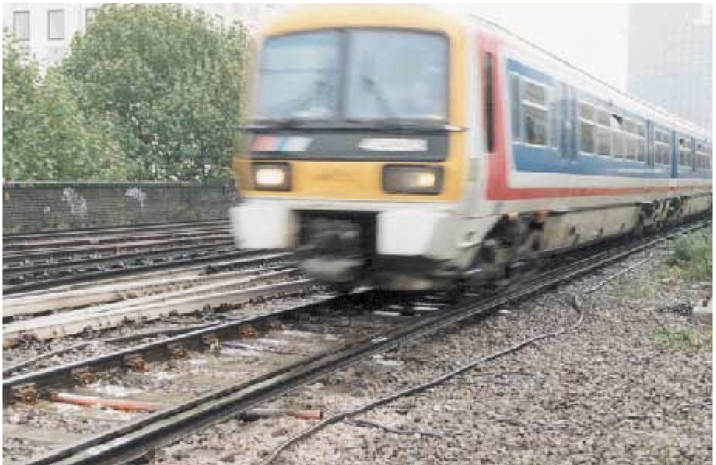
Completed Track in Service
