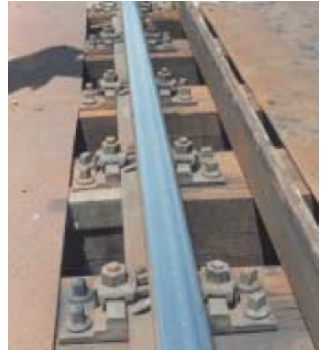
Fig 2: Original K type fastenings.
