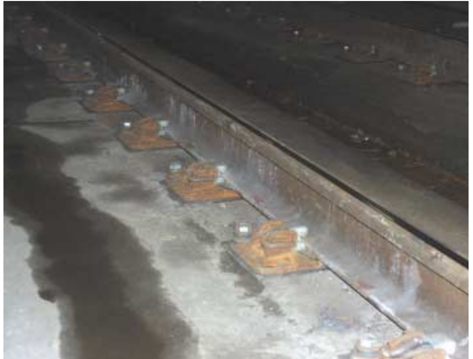
Pandrol FASTCLIP assembly.
