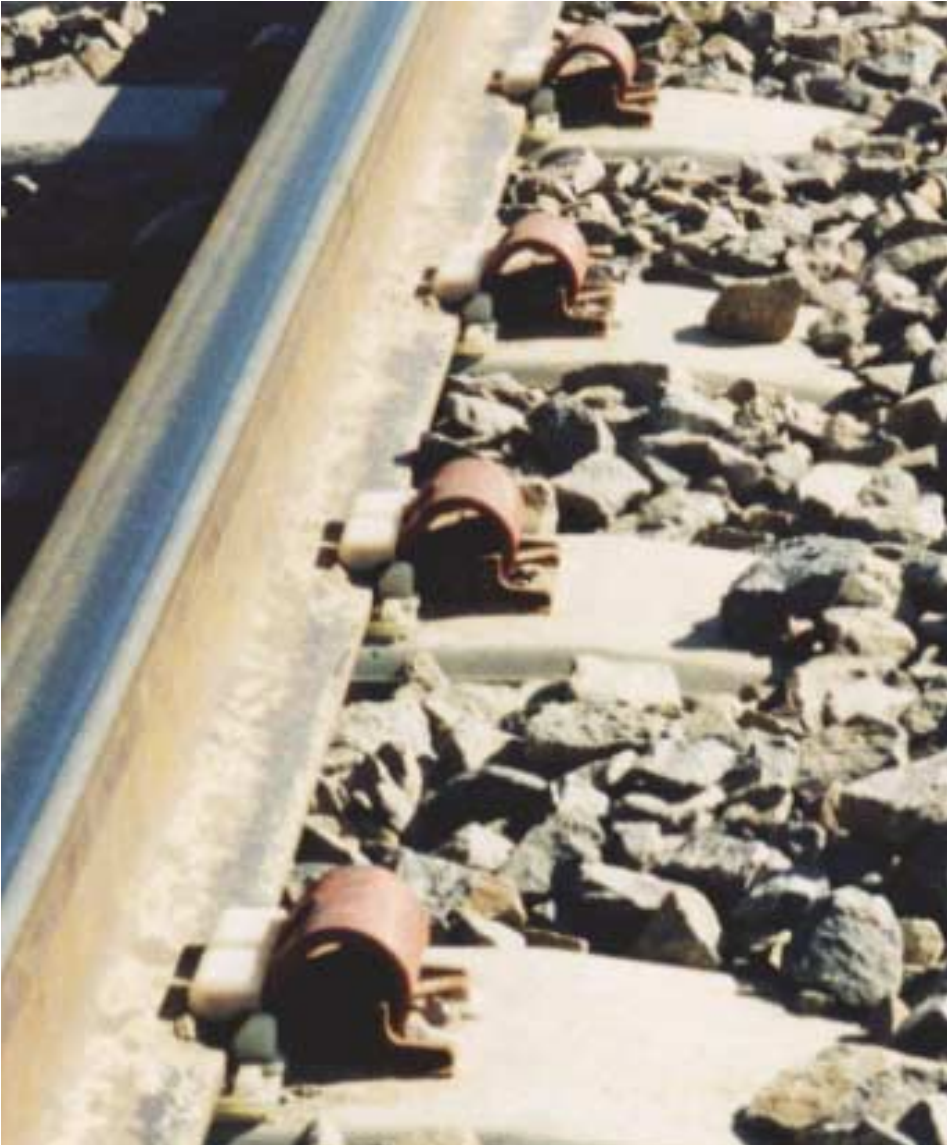
Left: SAFELOK III installed in track at Crawford Hill Nebraska.
