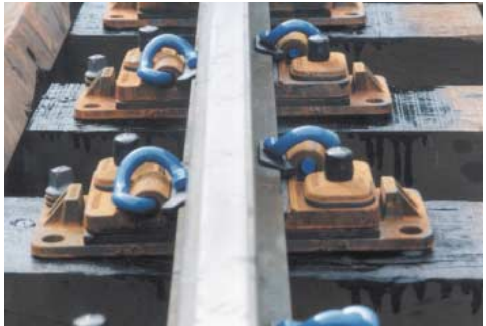
Fig 3: PANDROL VIPA Baseplates secured to timber sleepers.
