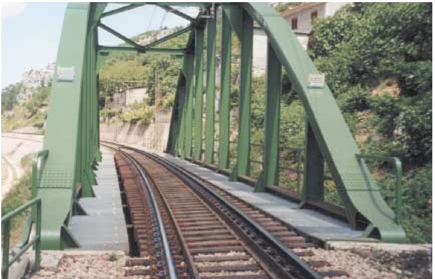
Fig 1: The Podpeč Steel bridge, showing proximity to adjacent houses.
