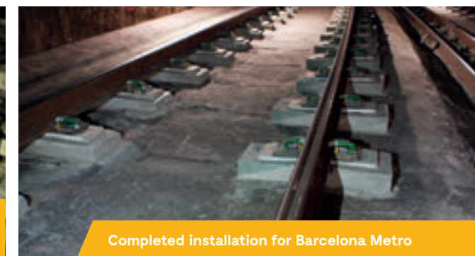
Lightweight concrete block delivered pre-assembled
