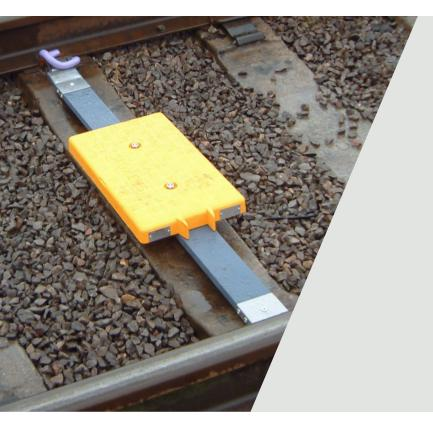
The Pandrol On-Sleeper Beam Balise Mounting System (BMS) is used to install balises (transponders) into track securely and efficiently.
