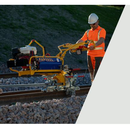
The Clip Driver CD200 IQ, the first machine in Pandrol's new IQ range, uses intelligent control systems to simplify operation. The new smart system can provide information on clips installed and number of operating hours, while also preventing incorrect use of the machine.
