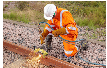
Oxy-propane cutting with gas cutting tools.
