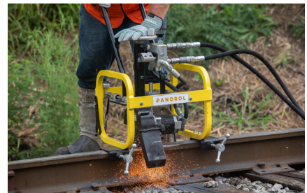
Grinding with head wash grinder.
