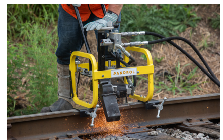
Grinding with head wash grinder.
