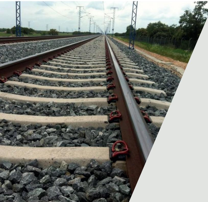
Pandrol SKL is a resilient, screwed-direct fastening for concrete sleepers. Simple, reliable and safe, it is a proven solution for ballasted track in many countries.
