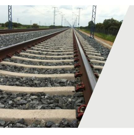
Pandrol SKL is a resilient, screwed-direct fastening for concrete sleepers. Simple, reliable and safe, it is proven solution for ballasted track in many countries.
