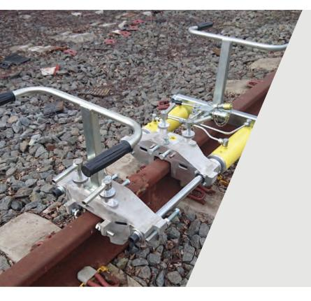
The Bi-Bloc Weld Shear EGH1/EGH2 is a hydraulic rail shearing machine designed to shear off excess metal after aluminothermic welding of Vignole rails. During aluminothermic welding, excess metal remains above the rail head. This was traditionally removed manually with a hammer and chisel. The Bi-Bloc Weld Shear automates this process and removes the risk of damaging the rail.
