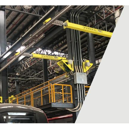
Pandrol's Retractable Catenary is a clever removable rigid catenary system designed to ease and secure maintenance operations on rolling stocks.
