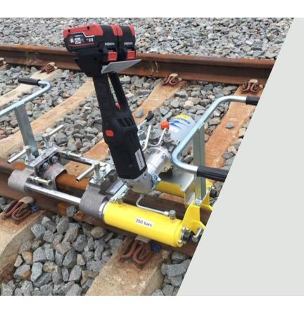
Pandrol's battery-operated weld shearing machines are designed for the easy removal of excess metal following an aluminothermic weld. The shearing process takes place after mould release.
