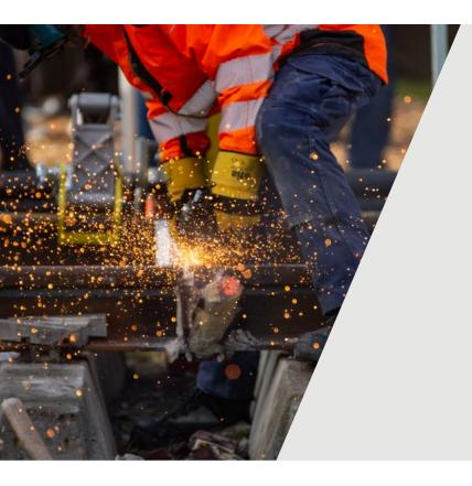
The fully portable and completely autonomous Pandrol Handheld-Grinder B-115-MTR is the perfect track side tool for finishing grinding work on all types of Vignole rails.
