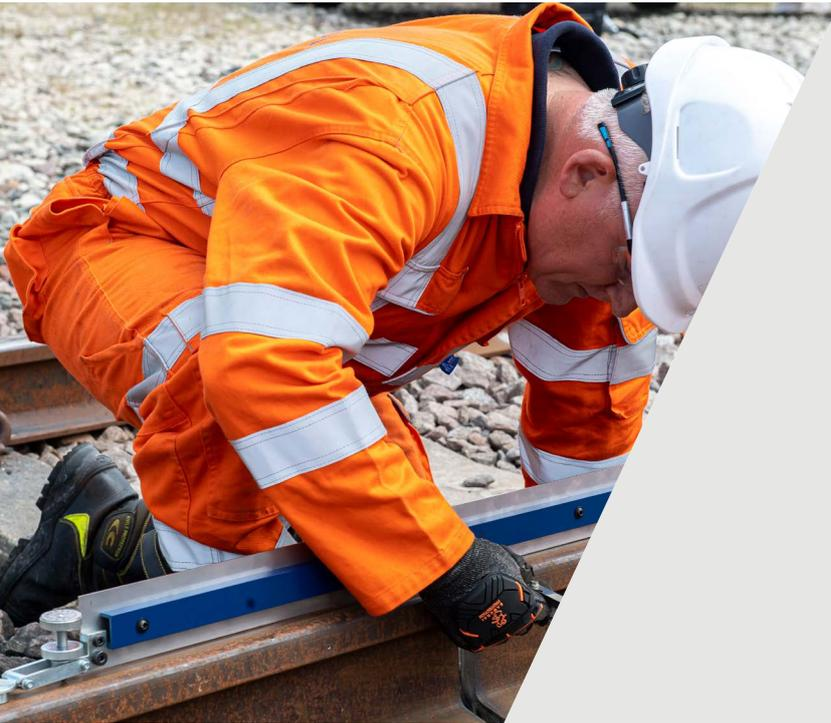
Pandrol Straight Edges are long-lasting, easy-to-use tools designed to ensure accurate alignment before aluminothermic welding takes place – and to check the grinding tolerance when it's complete.
