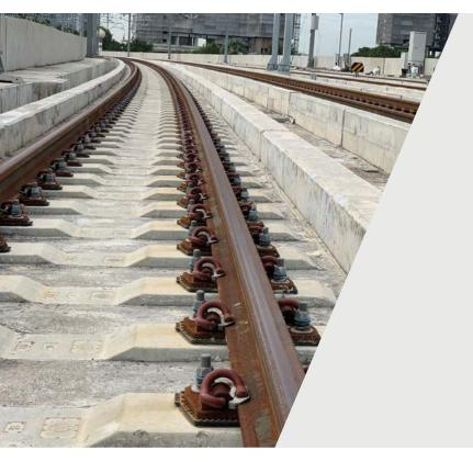
The DRS baseplate is a double-resilience e-clip fastening system that is ideal for use on non-ballasted tracks when ground-borne noise and vibration reduction are required. Originally introduced in the 1980s, today's evolution of the DRS baseplate is the trusted solution for metro, light rail and mainline slab tracks worldwide. Widely used on bridges, viaducts and in tunnels, it is suitable for all rail inclinations and rail types.
