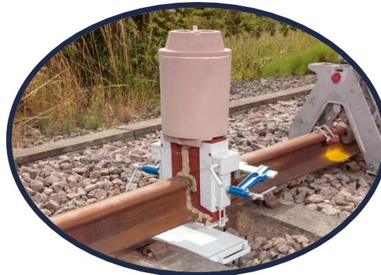
Aluminothermic Welding
