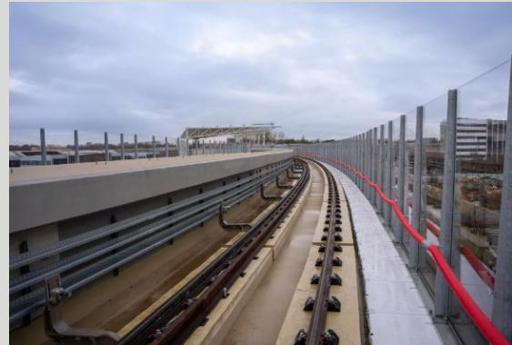
Pandrol also supplied, for the 14 km of the tunnel section, a total of 192,800 Safe Driven (SD) units, our pre-assembled high performance screwed fastening solution designed for concrete sleepers. This system was selected for its ease of installation and low maintenance requirements, while also helping to reduce distribution and handling costs during track laying.
