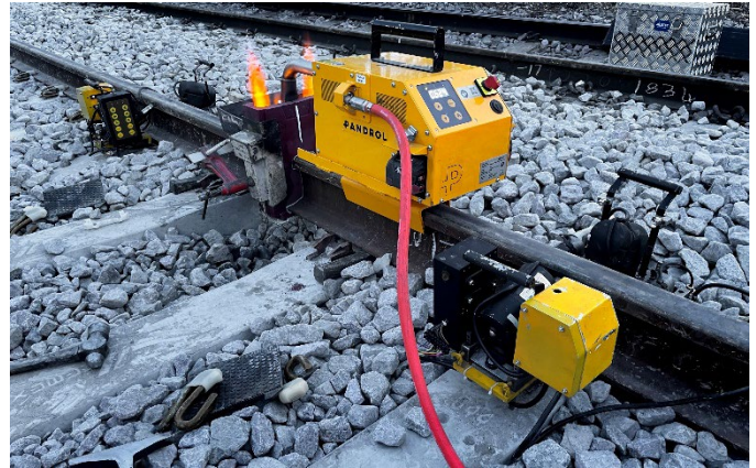
Fig.2: Welding on track with i+weld set up
